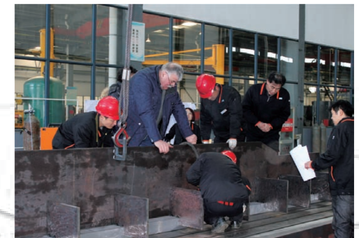
Steel Welding technology from Germany
